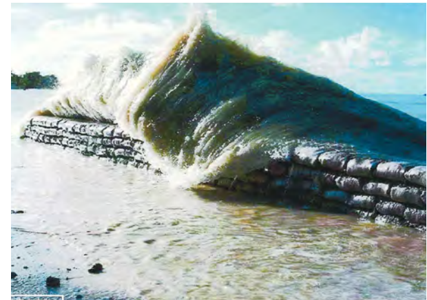
Waves overtopping roads caused by king tides
