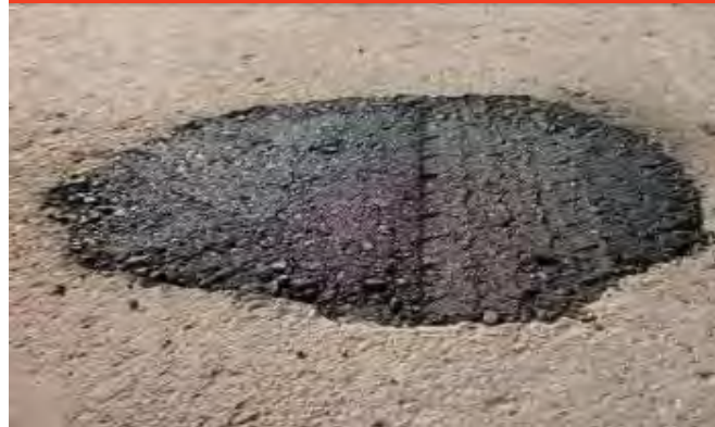
Conventional Cold Mix Asphalt
