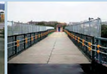
Temporary bridge for pedestrian walkway
