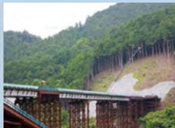
Temporary bridge for construction road
