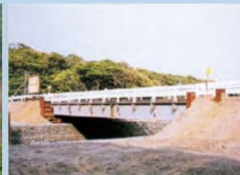
Emergency bridges in times of disaster
