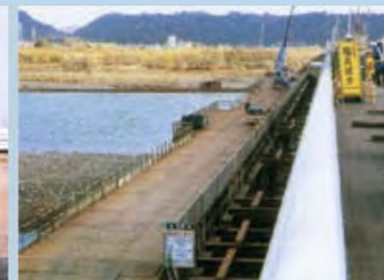
Temporary Jetties for cranes and other work
