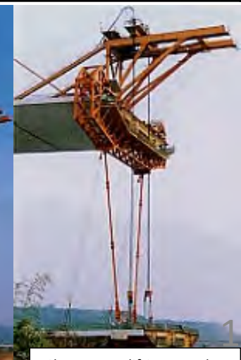
Change to a lifting traveler
