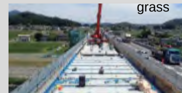
Bridge deck slab rehabilitation
