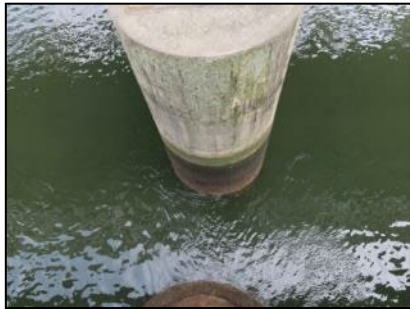
Site conditions (pier foundations)
