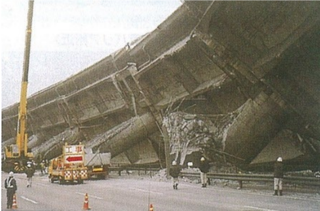
Damage from the Hyogo-ken Nanbu Earthquake
