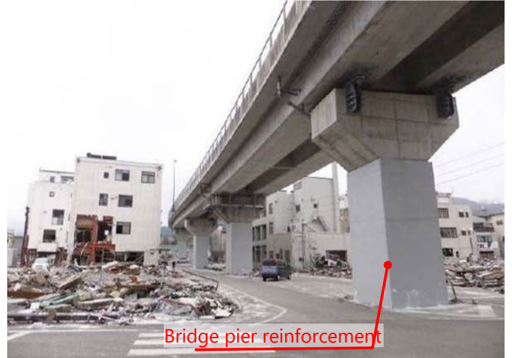
Situation of bridges after countermeasures
