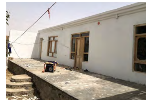
HOUSING AFTER REPAIRS
