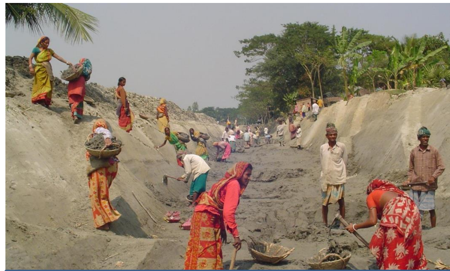
Canal digging Passage of flood water
