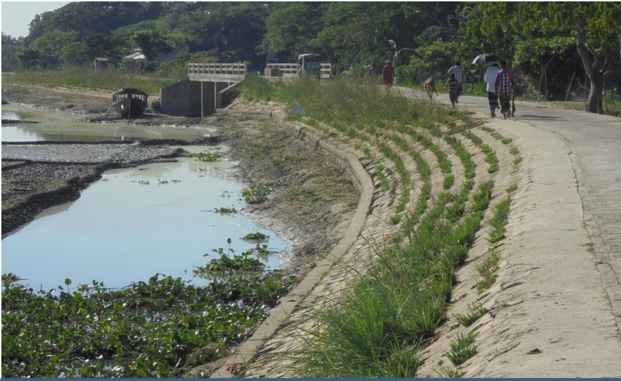
Protection of Road Embankment
