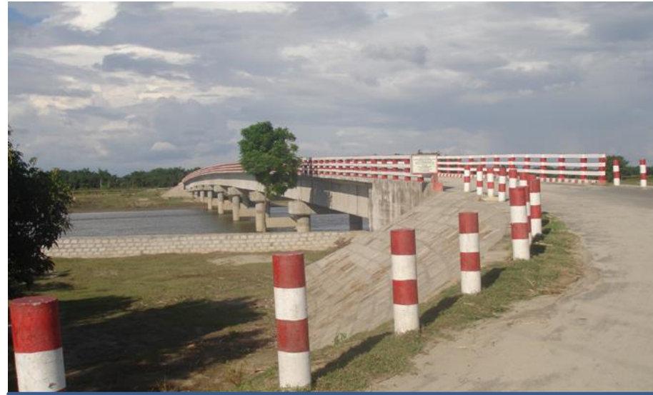
Protection of Bridge Approach
