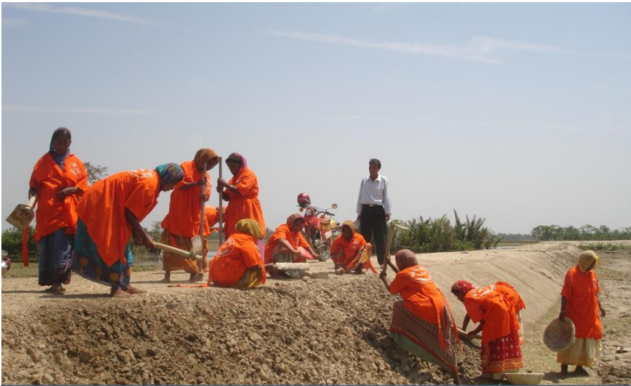
Raising the embankment height
