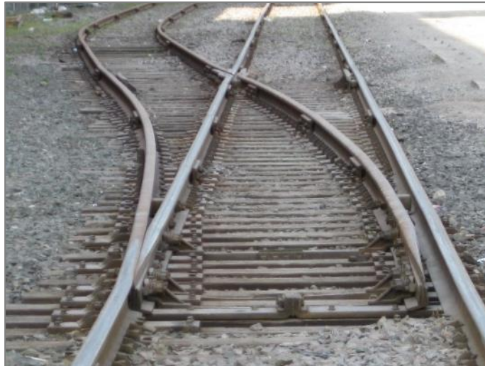
Figure 67: Switch and direction allowed
