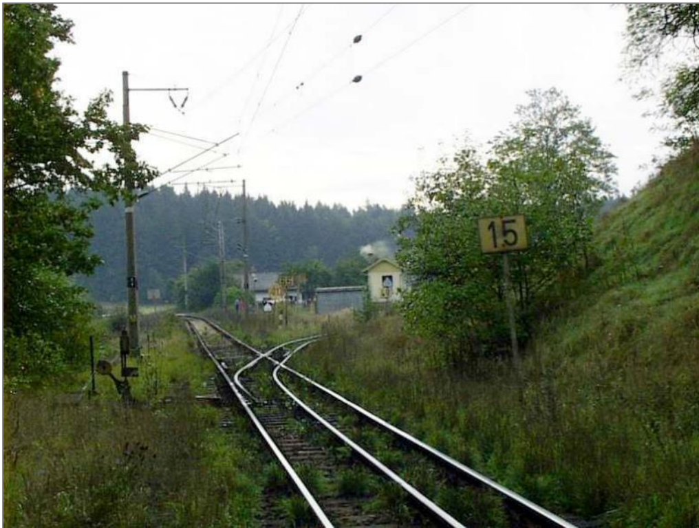
Figure 46: Two-gauge railway (metric gauge and standard) in Jindřichův Hradec (Czech Republic)
