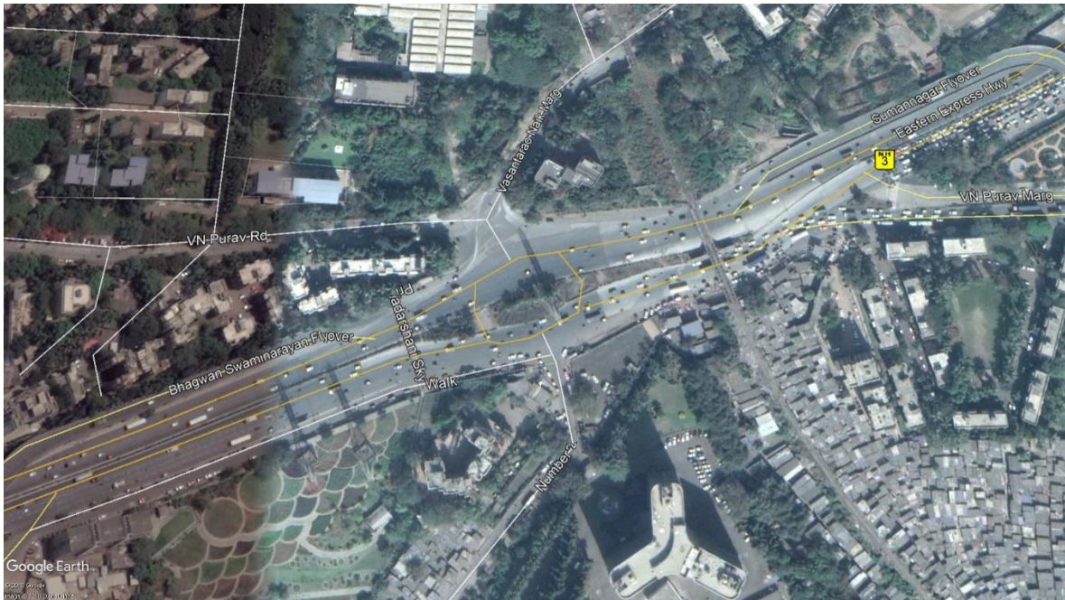
Figure 13: Google Earth satellite image of Priyadarshini Circle Intersection, accessed in September 2018
