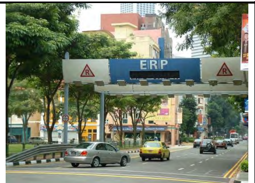
Singapore uses Electronic Road Pricing (ERP) that charges for driving on major roads during peak periods
