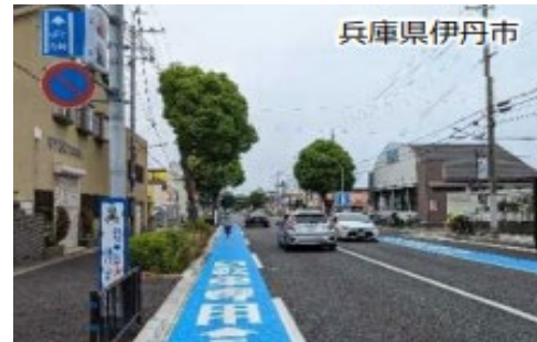
Installation of bicycle lanes
