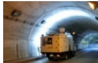
monitor deformation by laser scanning
