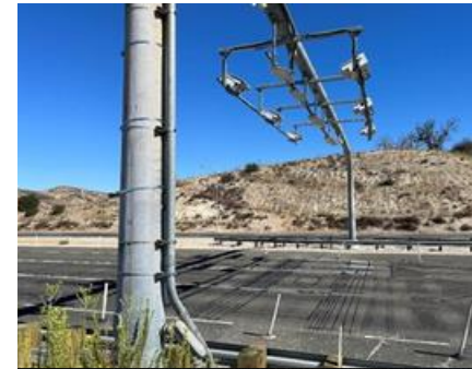
The system is able to weigh a vehicle while in motion automatically and continuously. Therefore, it can provide accurate vehicle weight information to enforcement and efficient enforcement implementation.
