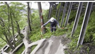
Inspection of unstable rock mass
