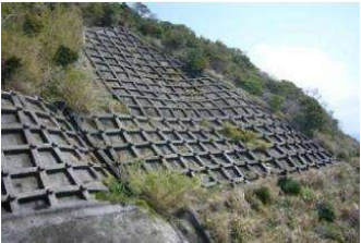
Crib Work + Anchor
