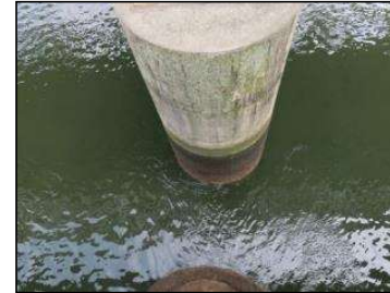
Site conditions (pier foundations)
