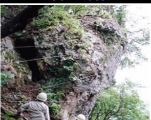
Inspection of existing prevention works
