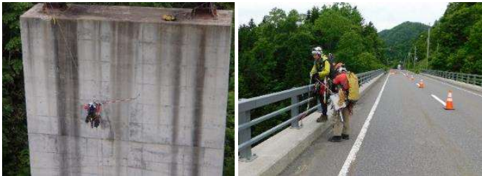
Rope access inspection status Traffic control is necessary
