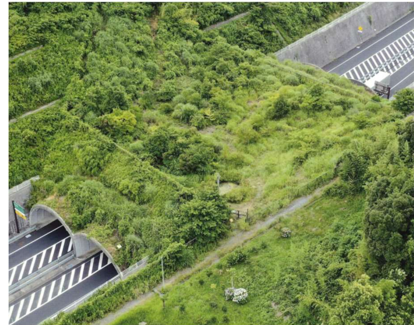
Mobara Animal Bridge Ken-O Expressway
