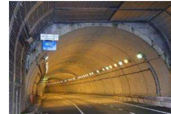
Mine entrance at the origin (downstream)
