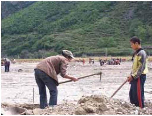
Fig.2 Villagers participating in housing construction.
