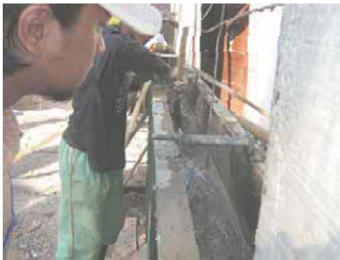
Fig. 1 Reconstruction using recycled rubbles
