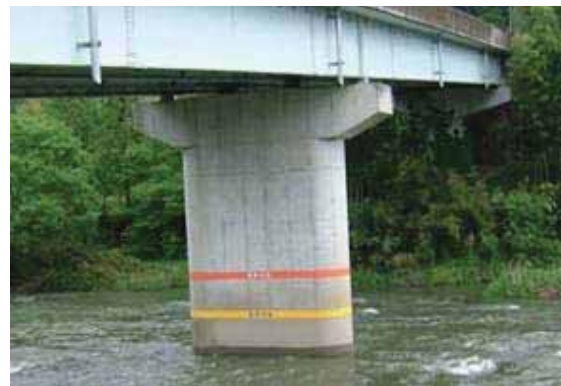
Fig.3 River water indicator for flood warning. Two marks differently coloured show the rise in water level.
