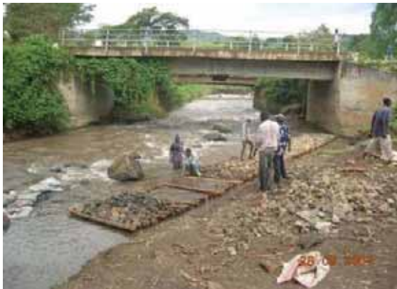
Fig.6 River improvement works using low-cost method.
