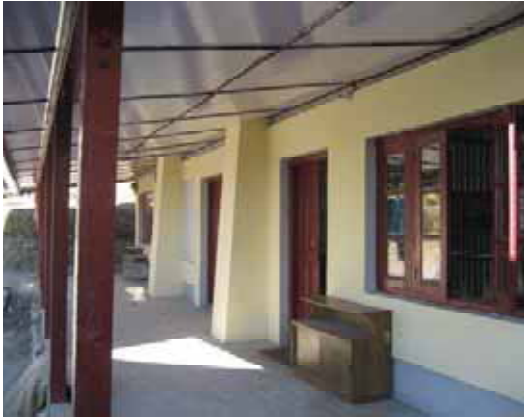
Fig. 3 Students' dormitory after the retrofit
