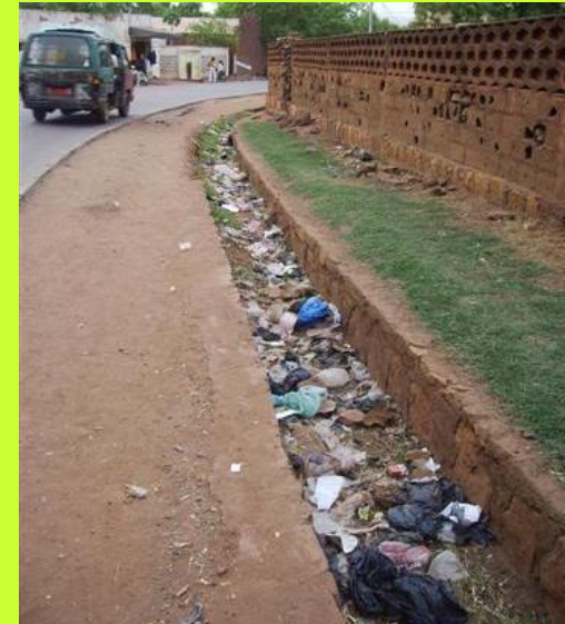
Waste blocking a storm drain, Bamako, Mali
