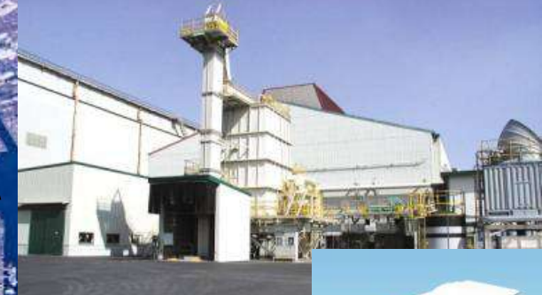
Plastic Recycling Plant (Blast Furnace, Mold Panel Production Plant)/E-waste Recycling Plant (JFE Group)
