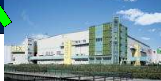
Nonrecyclable Paper Recycling Plant (Sanei Regulator Inc.)
