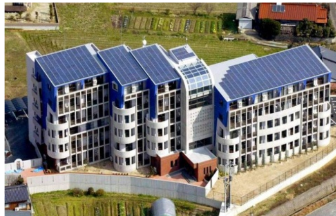
Rented-type eco-apartment house with photovoltaic power generation (First in Japan)
