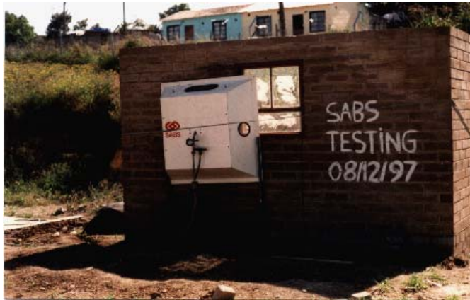
24-hour rain penetration test
