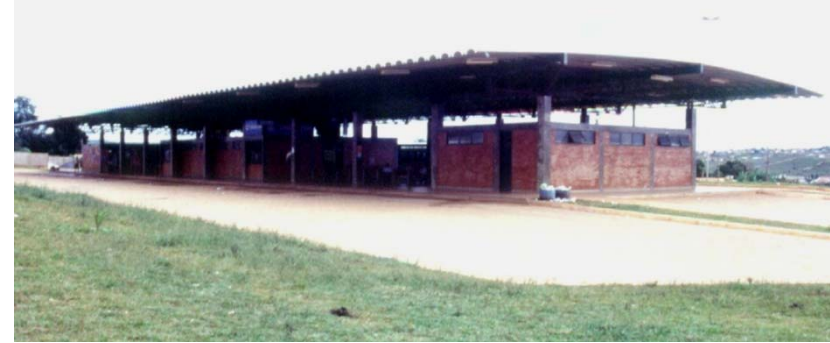
Construction of a new bus station in the new (displaced) City Centre)
