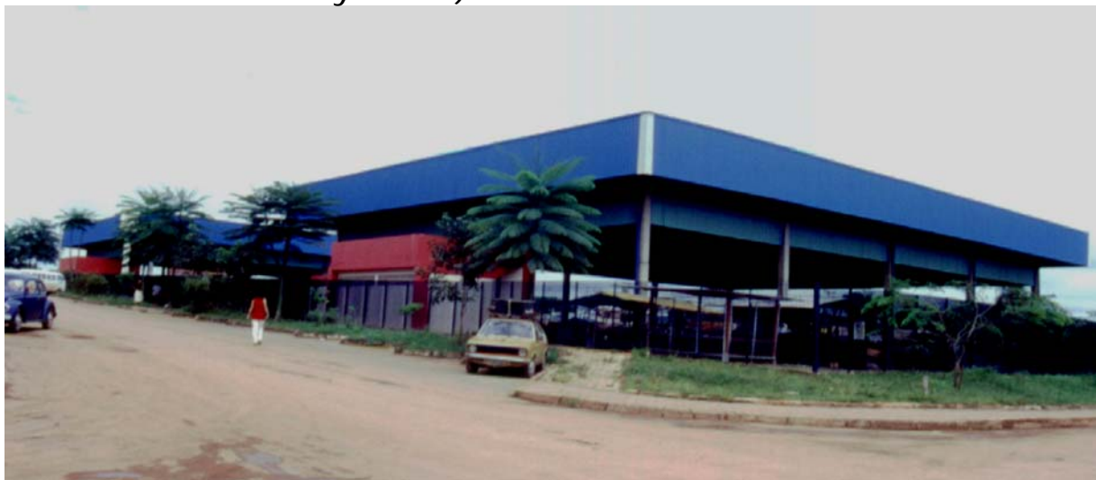
Construction of the Covered Market in support to small businesses (hawkers) Note: Planting trees along the main streets (in collaboration with local schools)
