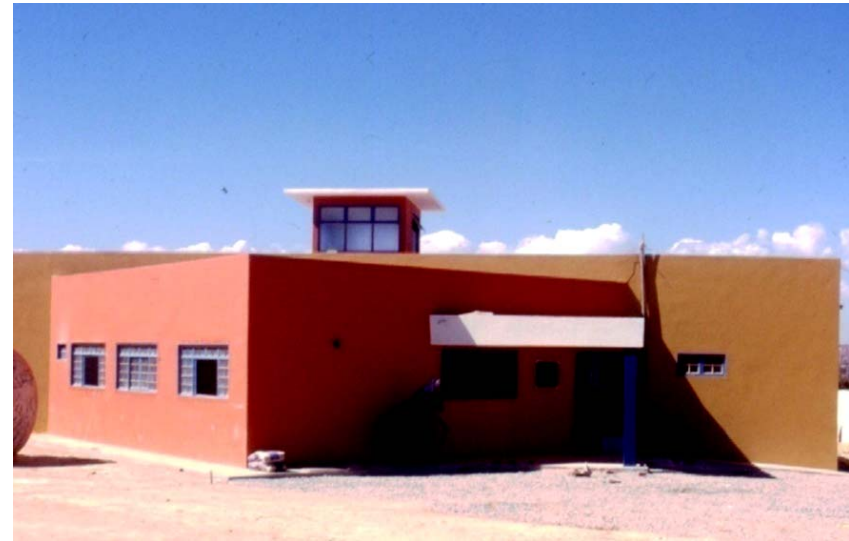
Construction of the Penitentiary
