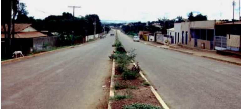
The new municipal road system (with storm water drainage and wastewater sewer systems)
