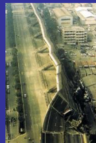
Collapsed Hanshin Expressway Kobe Route
