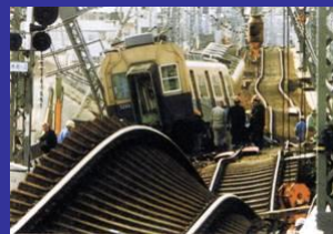
Railway train tracks were mangled
