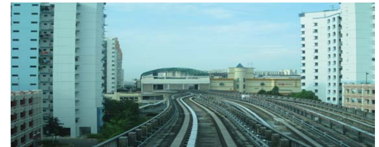
Singapore's LRT System developed around purpose-built-communities in which residential, shopping, education, public services and workplaces are all co-located. Photo: Lloyd Wright
