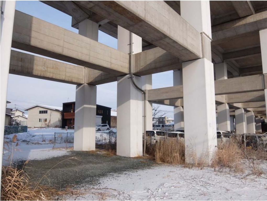
Steel Jacketing (Tohoku Shinkansen, Morioka city)
