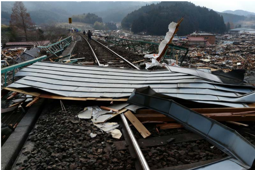
Debris on railway (South-Rias Line)
