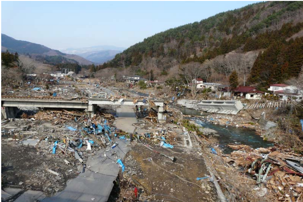
Washed away Bridge (South-Rias Line)
