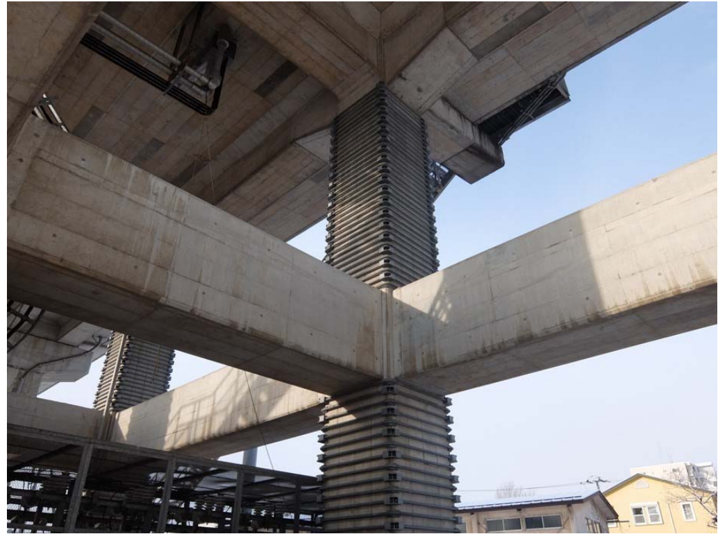
Rib-bar retrofit (Tohoku Shinkansen, Morioka city)
