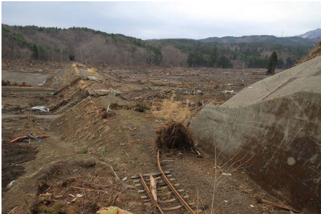
Just after the earthquake (North-Rias Line)
