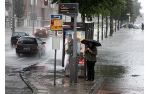
Excess stormwater on the street
