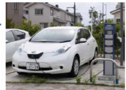
Two EVs are reserved. In case of an emergency, the V2H system supplies electricity to the assembly room, etc.
