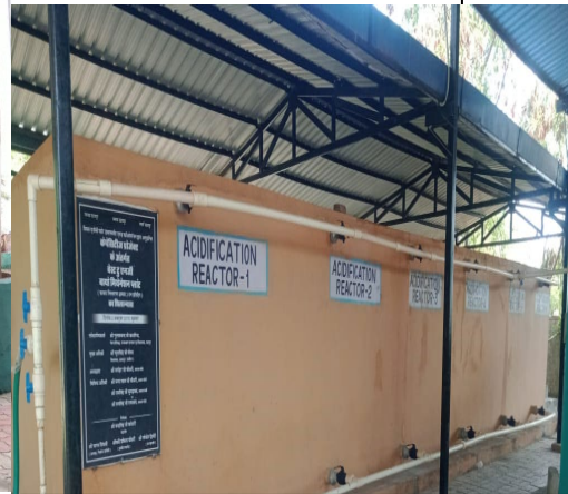
3. Waste slurry is pre-treated; addition of 200 kg/d of sewage sludge
