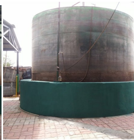
4. Pre-treated slurry is fed into bio-digester
