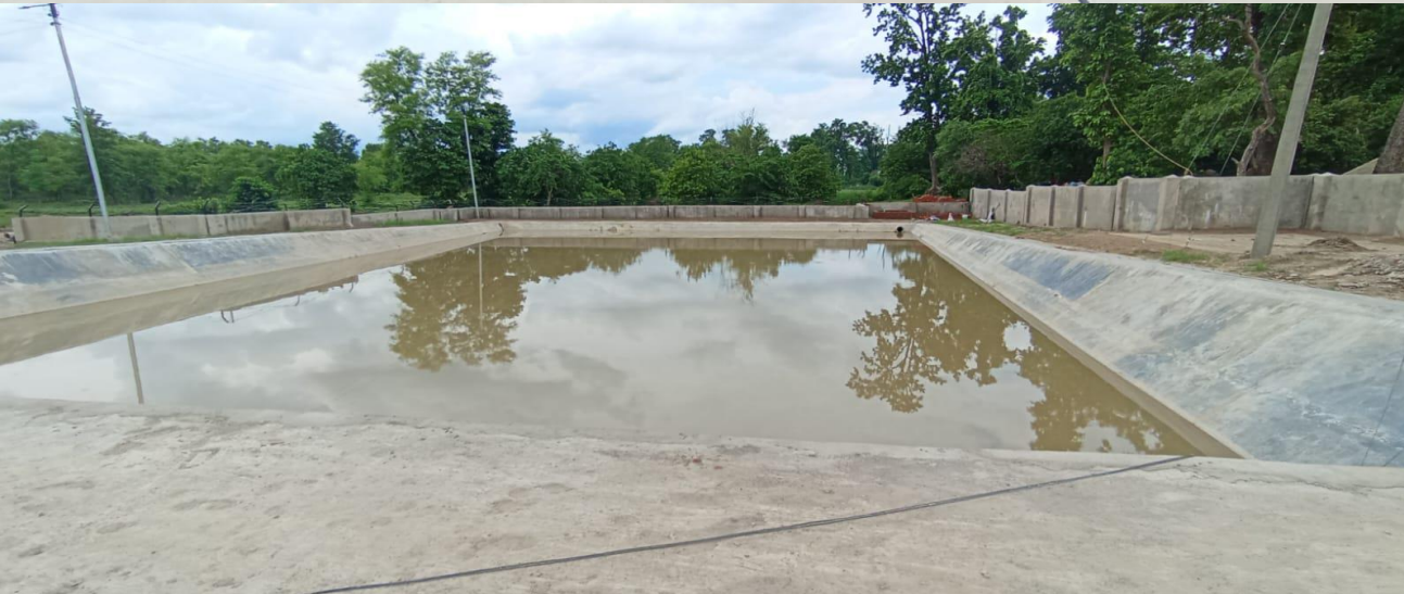
3. Leachate collection tank
