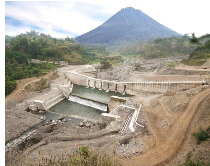
Erosion control dam in Mount Merapi, Indonesia
