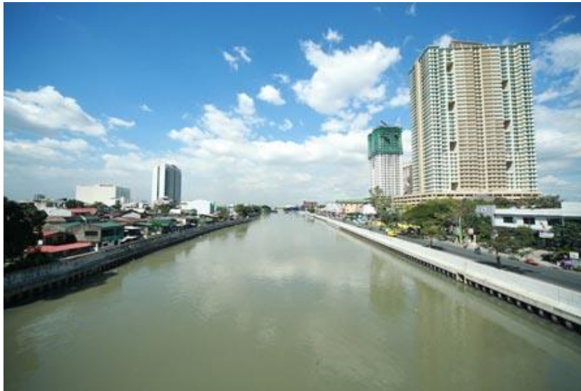
Pasig-Marikina river channel improvement project, the Philippines
