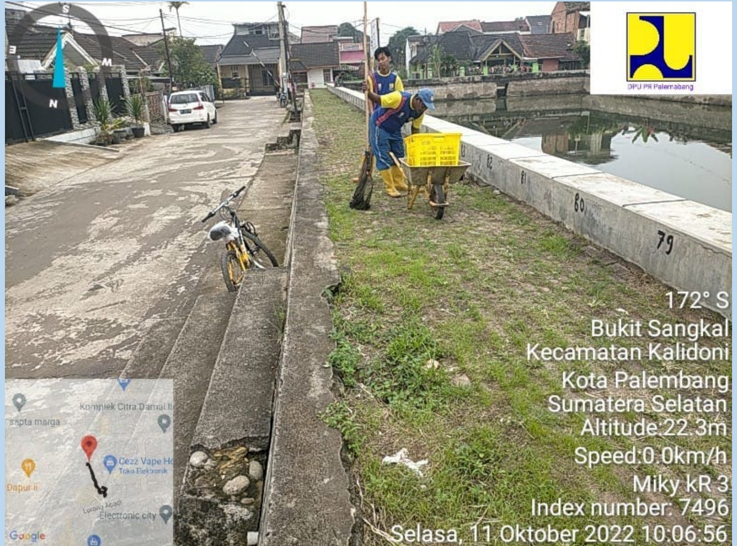
Location: Citra Damai Retention Pump
