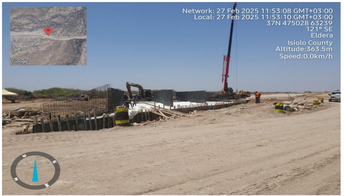
Triple cell box culvert
