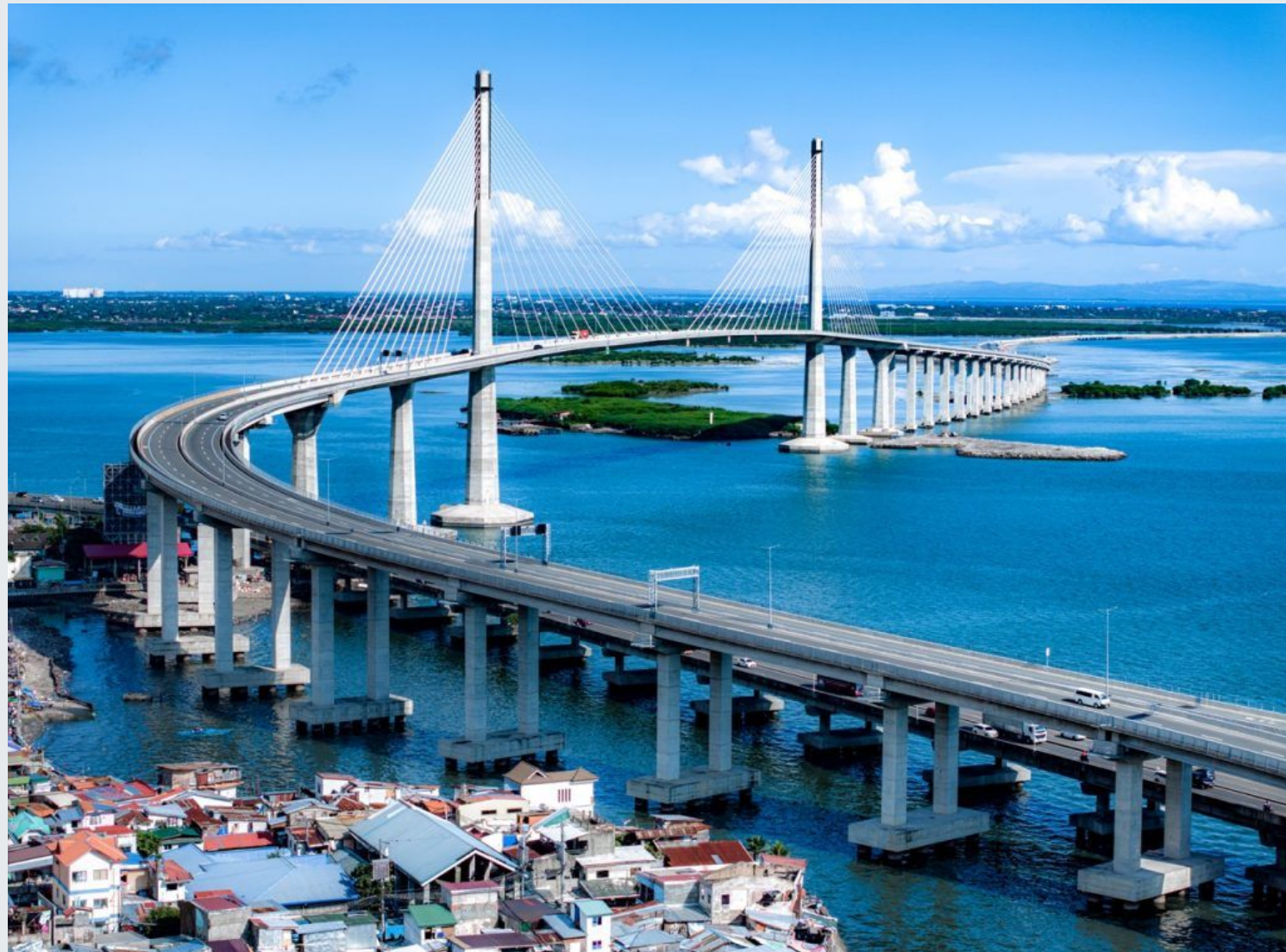
CEBU CORDOVA LINK EXPRESSWAY (CCLEX)
