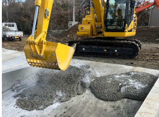
Granulate leftover/ returned concrete
