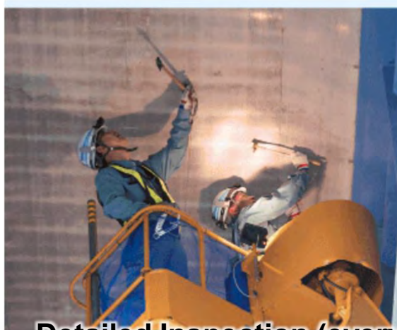
Detailed Inspection (every 5 years: Close-up Visual/ Sounding)
