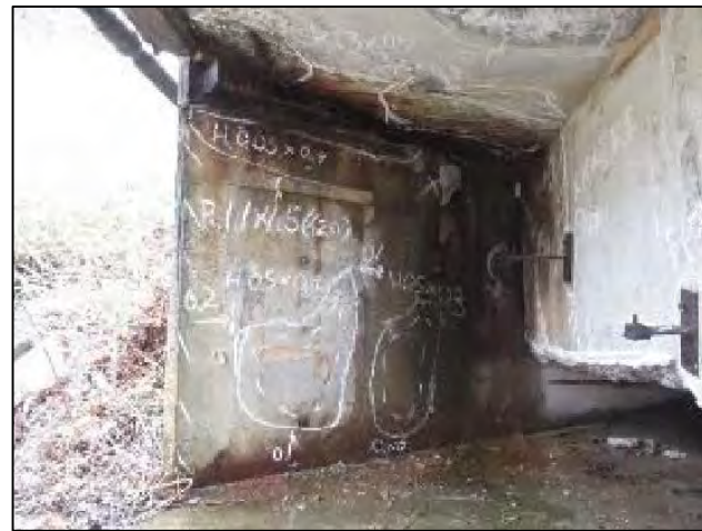
Girder ends and Bearings (46% of CS-III)
