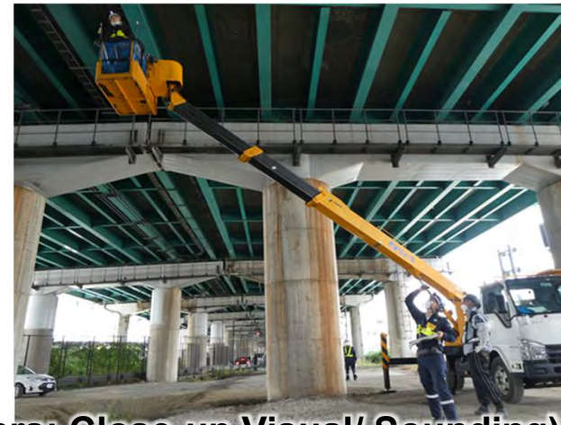
Detailed Inspection (every 5 years: Close-up Visual/ Sounding)
