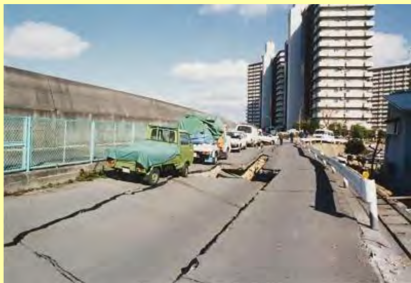
Damage to seawalls due to the earthquake
