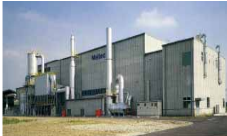
Bottom ash recycling facility
