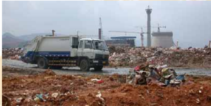
Incinerator construction in Kunming, viewed from the landfill
