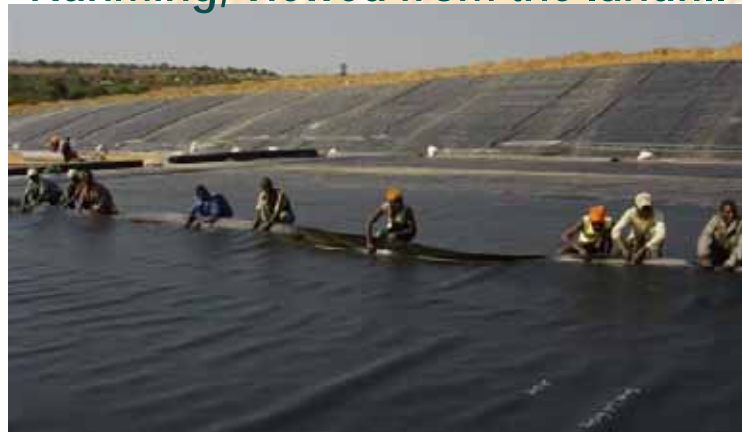
Landfill construction in Lusaka
