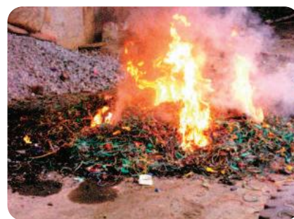
Removing plastics from coated copper cable, by using fire, which generates air pollution, including harmful dioxins.
