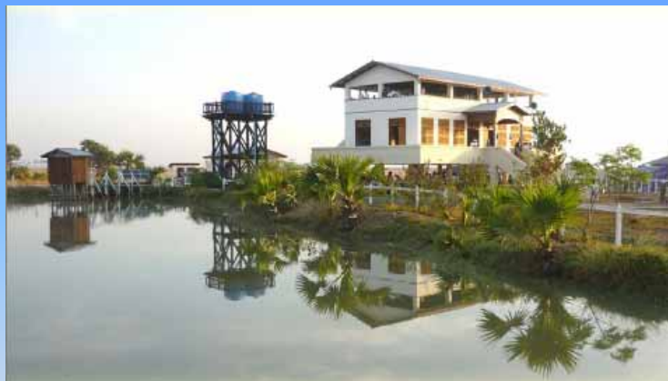
Solar Lighting and Solar Water Pumping Project at Auk Pyun Wa Village
