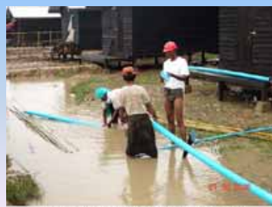
Laying Water Pipes to Individual Homes
