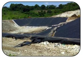
Photo 2 A cell of the landfill is being covered with clay and geosynthetic liner system during its construction.
