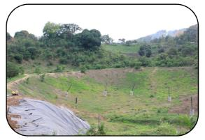
Photo 4 The disposed wastes are covered with geotextile instead of compacted soil. This was taken one month after the SLF operated in April 2015.
