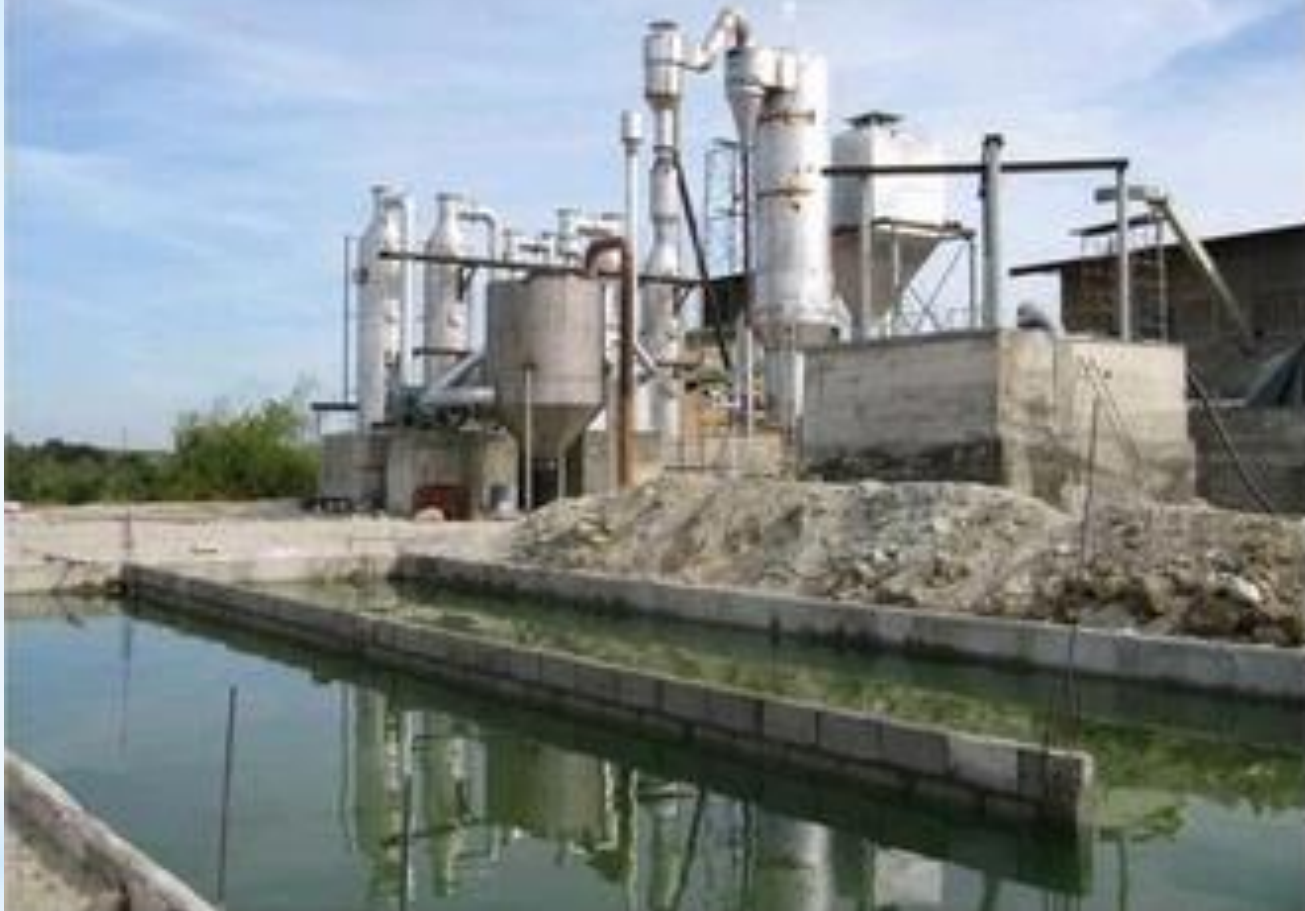
Biomass Gasification Power Plant System in Chongqing, PR China
