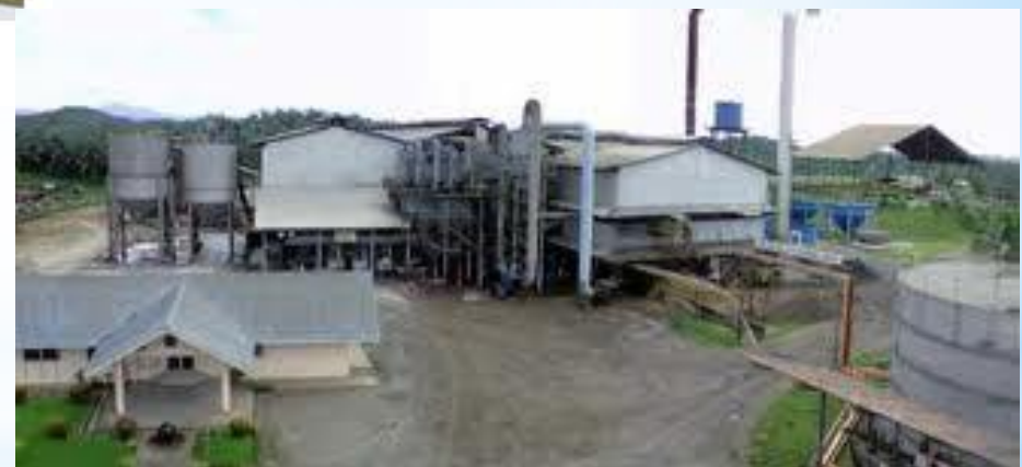
Palm oil mills in Malaysia use biomass to power itself in the form of combined Heat and Power usage
