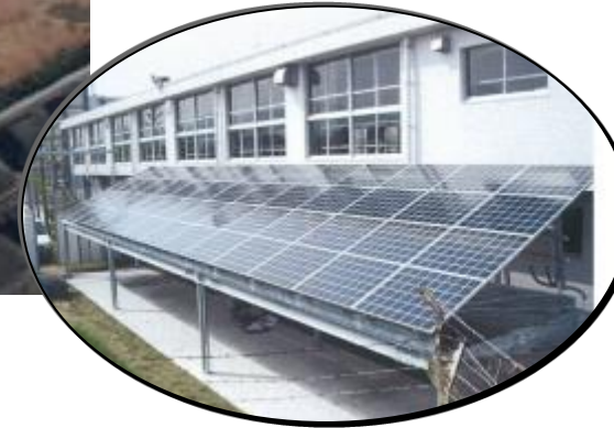
R&D on recycling technologies for solar power systems
