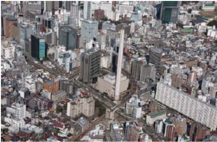
Shibuya Incineration Plant Constructed in 2001
