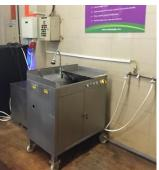
Food waste collection for co-digestion with used water sludge at demo facility
