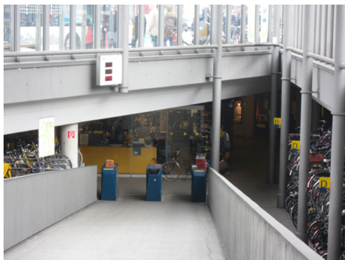
Figure 30: Underground bike parking station at Muenster main railway station..
