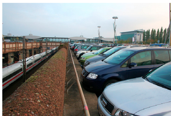
Figure 29: A Park & Ride facility at Kassel, Germany. Photo: Schmid, 2010.
