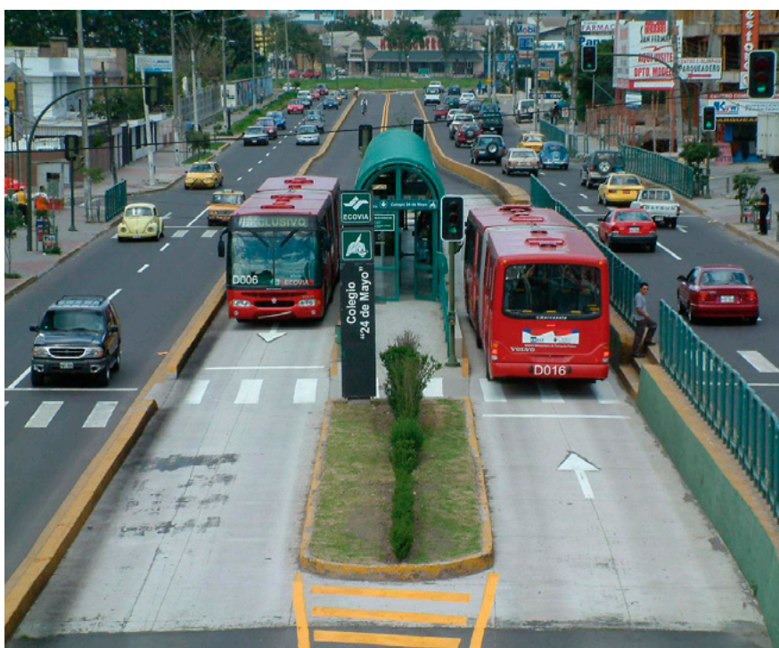
Figure 6: BRT-Stop in Quito, Ecuador. Photo: GIZ, BRT Standard 2013
