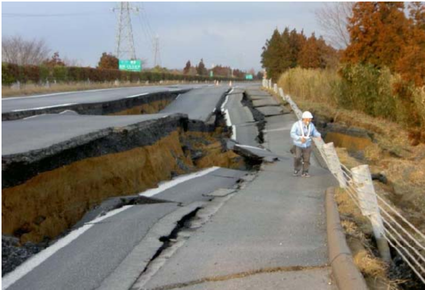
Soon after the earthquake, on March 11, 2011
