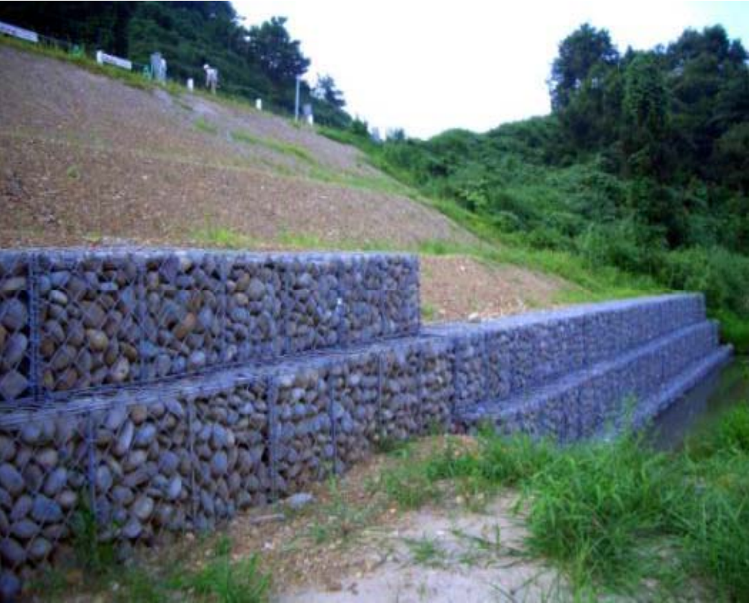
Gabions installed
