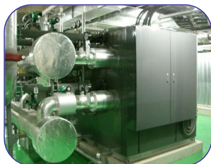
Ice thermal storage system
