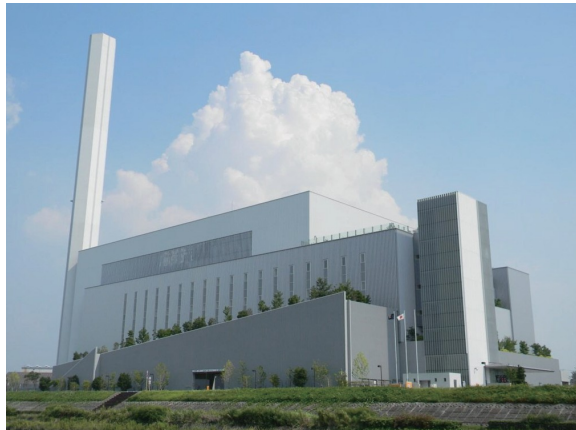
Waste incineration factory Waste to energy
