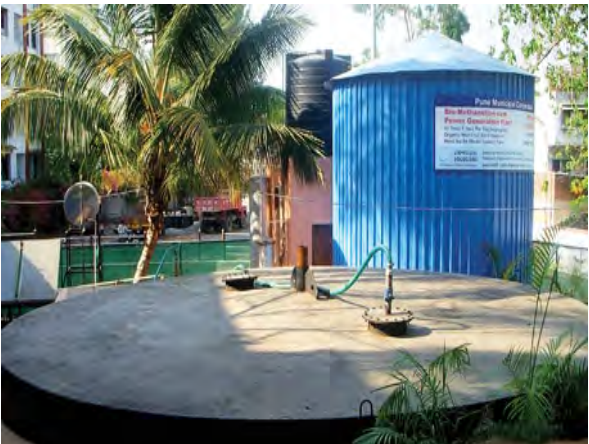
Biogas Plant in Pune
