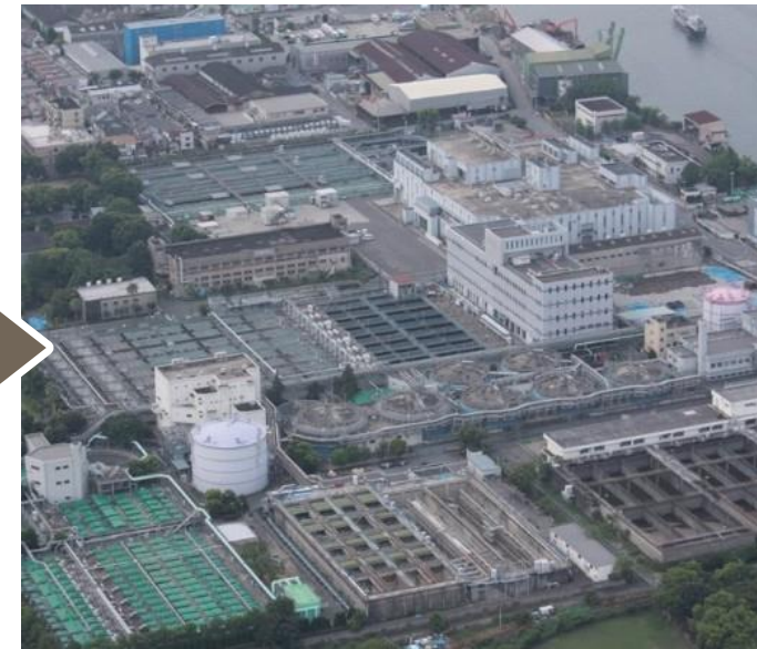
Tsumori Sewage Treatment Plant today
