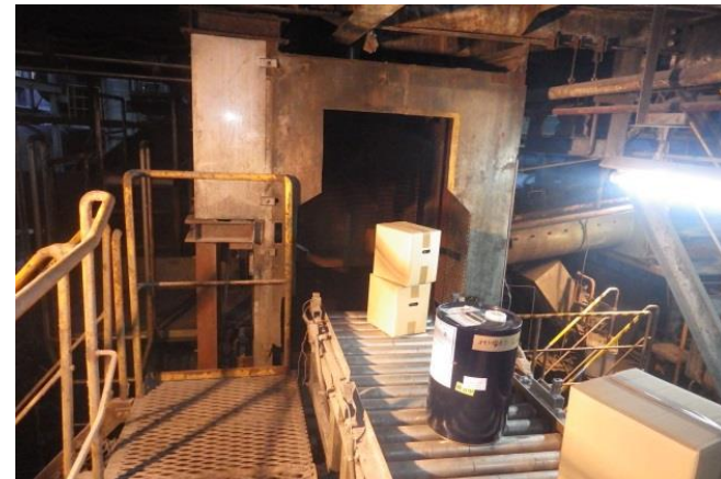
Direct Feeding into the kiln to prevent contact of wastes
