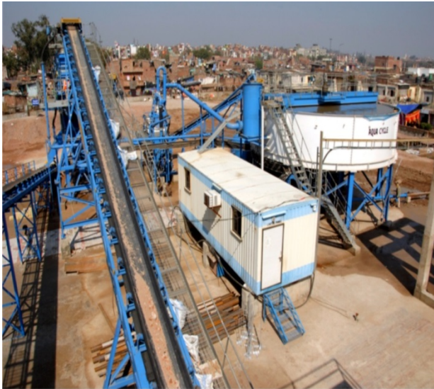
Crushing units at Burari C&D waste recycling plant Picture credits: IL&FS Pvt Ltd
