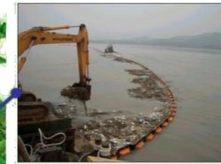
Isolation fence installation
